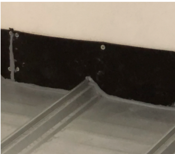
Figure 3: Sealant applied at the joints between the roof tile and EVA.
