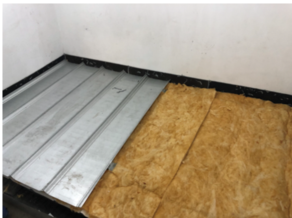
Figure 11: Installation of the upper zipper roof tile.
