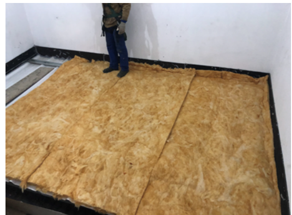
Figure 10: Installation of the glass wool.
